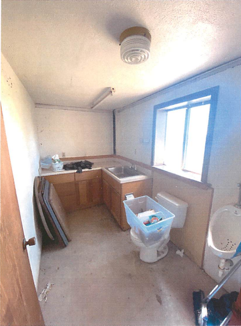
Picture 4: Bathroom space
